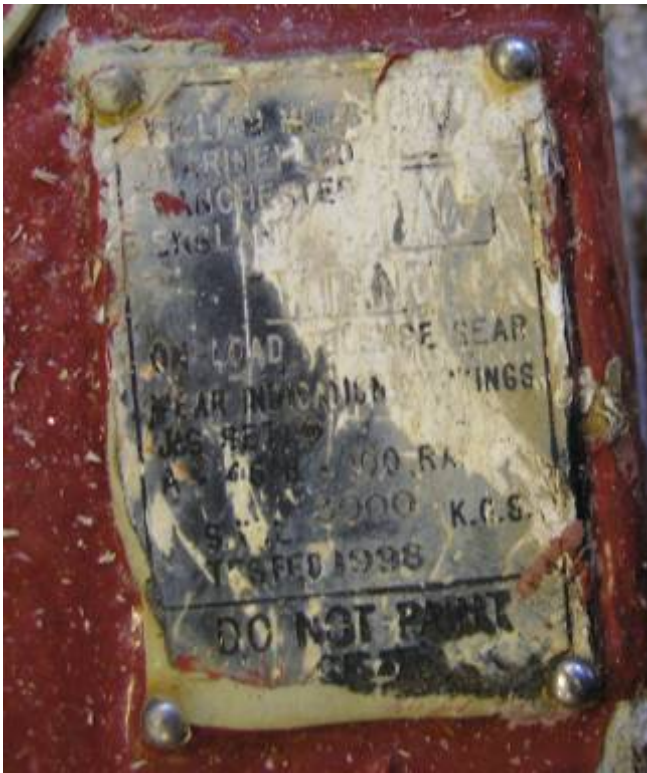
Figure 3: Manufacturers - Sign Plate of forward hoisting hook
