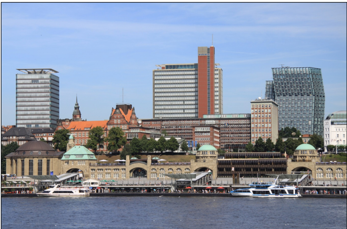
Figure 1: The BSU's offices in the BSH 1 building in Hamburg. The piers are visible in the foreground. In the background are the so-called 'Dancing Towers' to the right and the Astraturm to the left.
