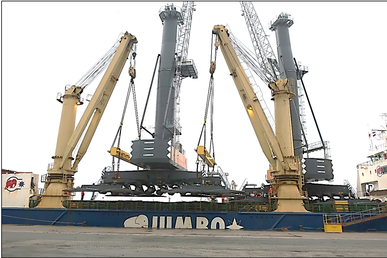
Figure 9: Crane 2 being tandem lifted 11
