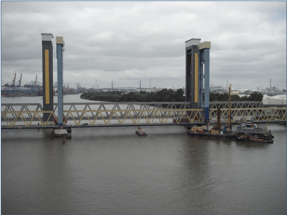
Figure 14: The Kattwyk bridge, which was also lowered at the time of the accident. 23
