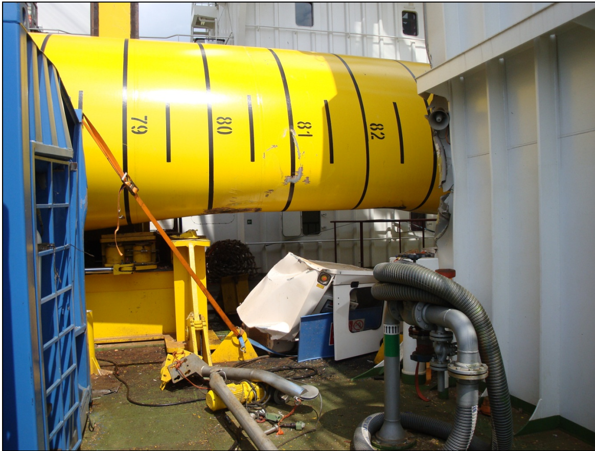
Accident involving the shipboard crane belonging to the wind turbine installation vessel WIND LIFT 1, BSU Investigation Ref.: 215/10, published on 01/06/2011 Source: BSU
