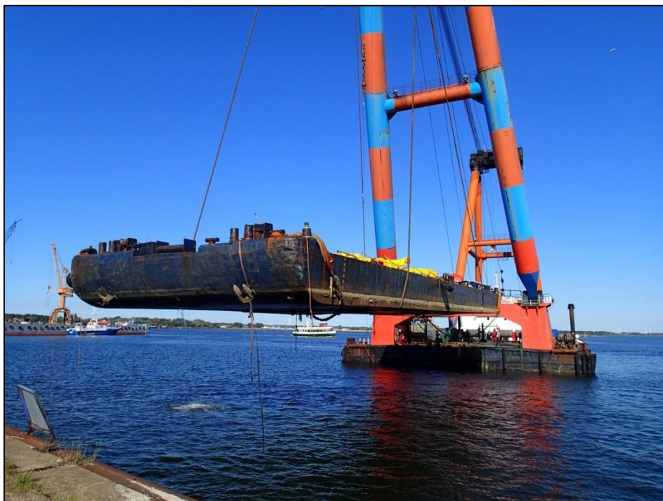
Salvage of the foundered pontoon
