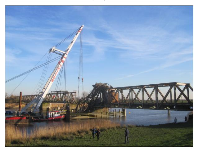
On 3 December 2015, the cargo ship EMSMOON, proceeding to sea from Papenburg, collided with the closed section of the Weener railway bridge. A large part of the bridge was destroyed, while the damage to the ship was less severe.
