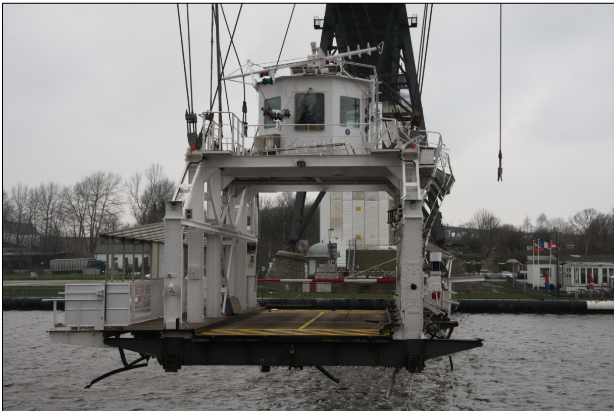
Damaged transporter bridge
