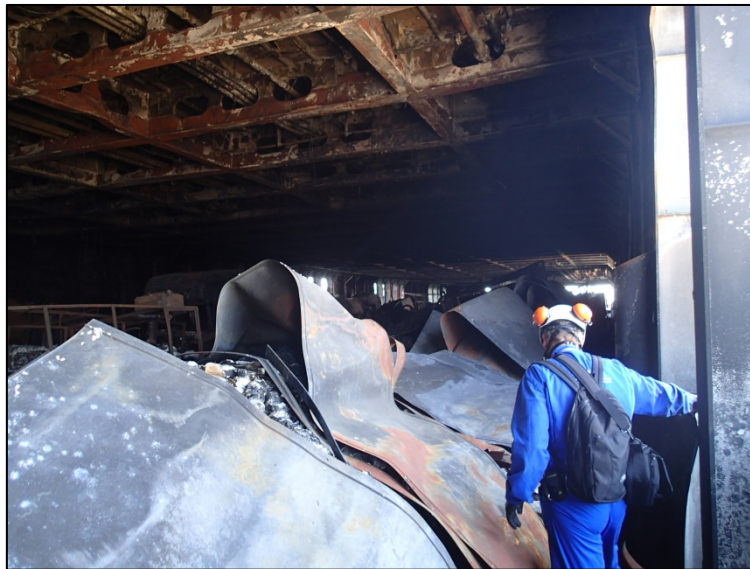
View into one of the ferry's cargo decks
