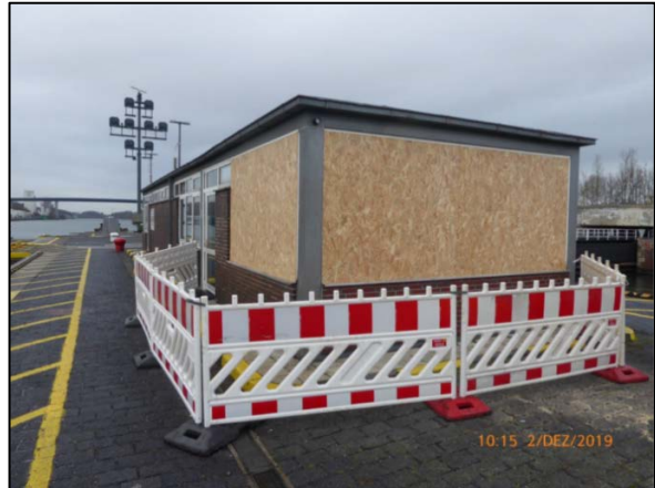
Figures above and below left: Damage caused by the rebounding line (Source: WSP) Figure below right: Linesmen's cabin provisionally sealed (Source: WSP)
