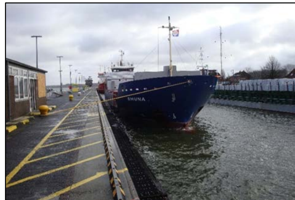
Figure to the right: Similar ship made fast in the lock with the linesmen's cabin on the left-hand side (Source: WSP)
