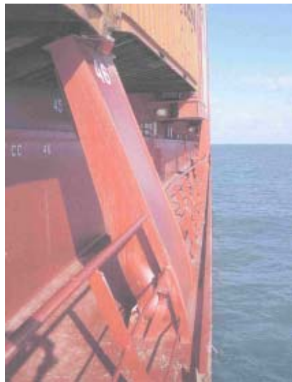
Picture 6: damage photo 2
