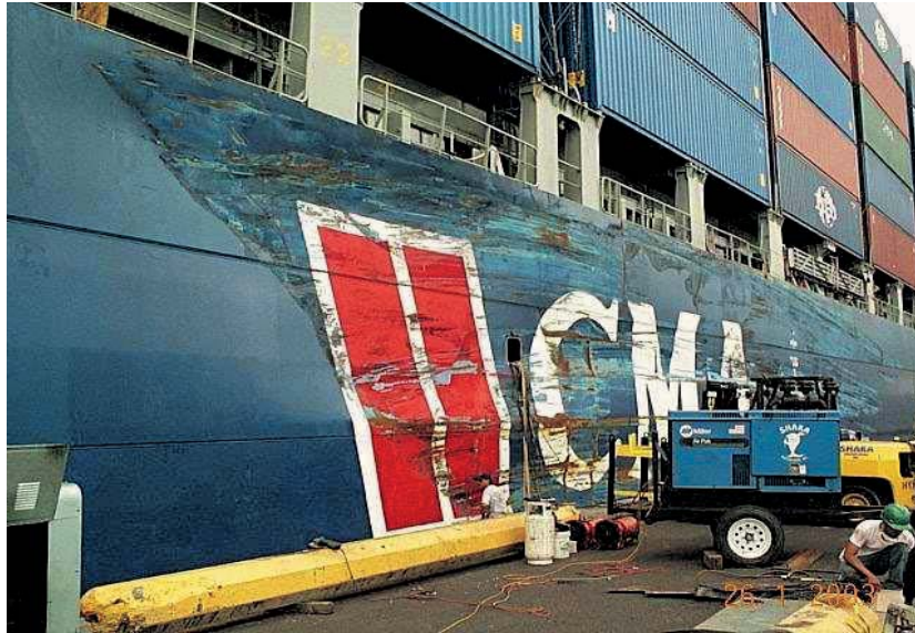
Figure 3, Emergency repair to the Container M/V "VILLE D'ORION" at the Pier in Honolulu
