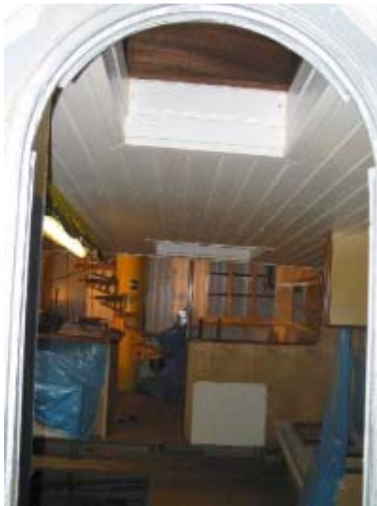
Photo 11, Front bulkhead door and skylight
