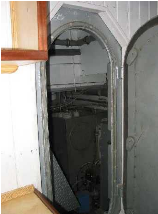
Photo 10, Aft bulkhead door
