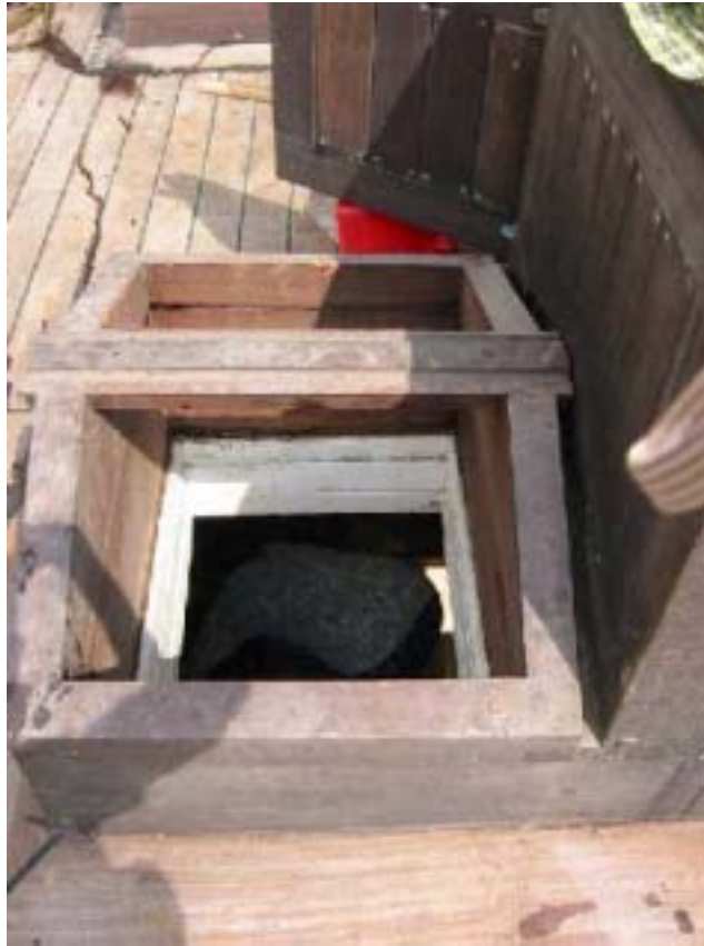
Photo 20, Open skylight after the salvage
