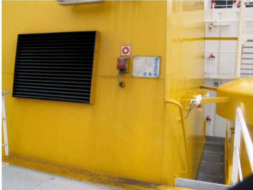
Figure 3: Inert gas outlet
