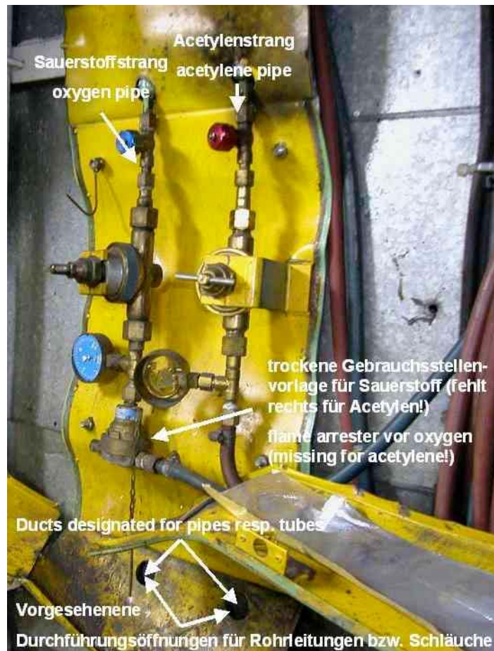
Figure 10: Detonated fitting cabinet (view 2)
