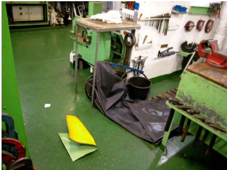
Figure 6: Curtain ripped away and heavily deformed fitting cabinet door
