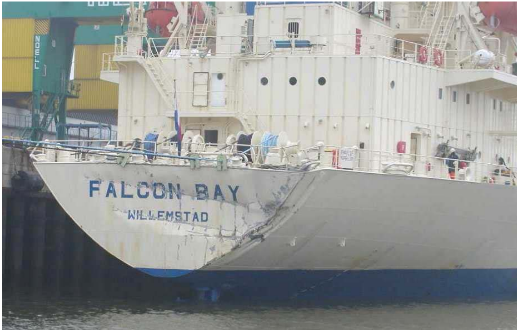
Figure 16: Photo of the damage 2
