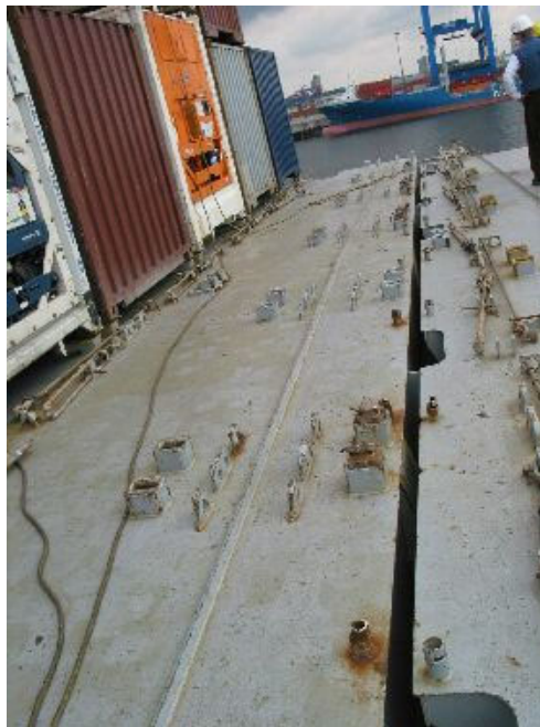
Figure 9, Catwalk between Hatches 1 and 2
