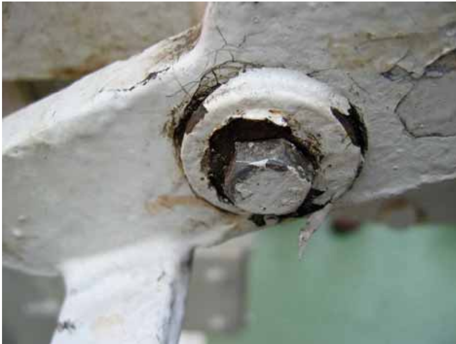
Figure 12: Safety bar, fastening screw
