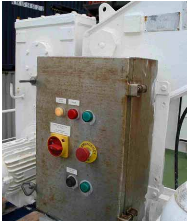
Figure 9: Dead angle behind the operator's location
