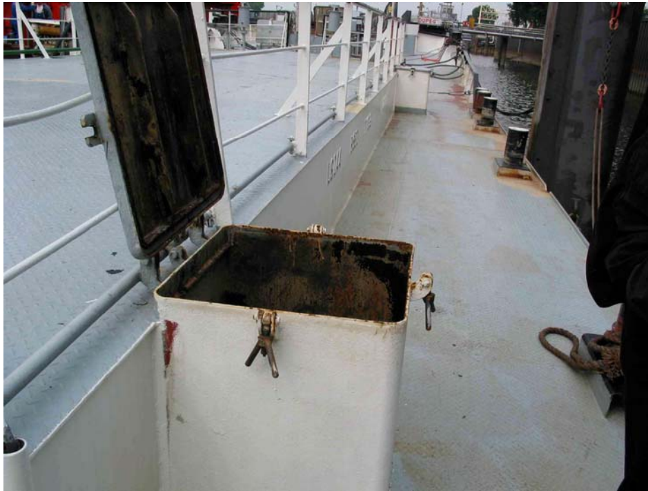
Figure 7: Entrance hatchway, wing tank
