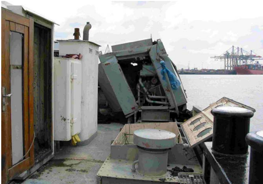
Figure 10: Deformed port Schottel drive housing
