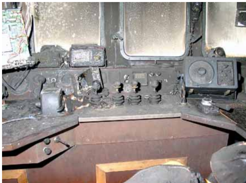
Figure 8: Wheelhouse looking forward
