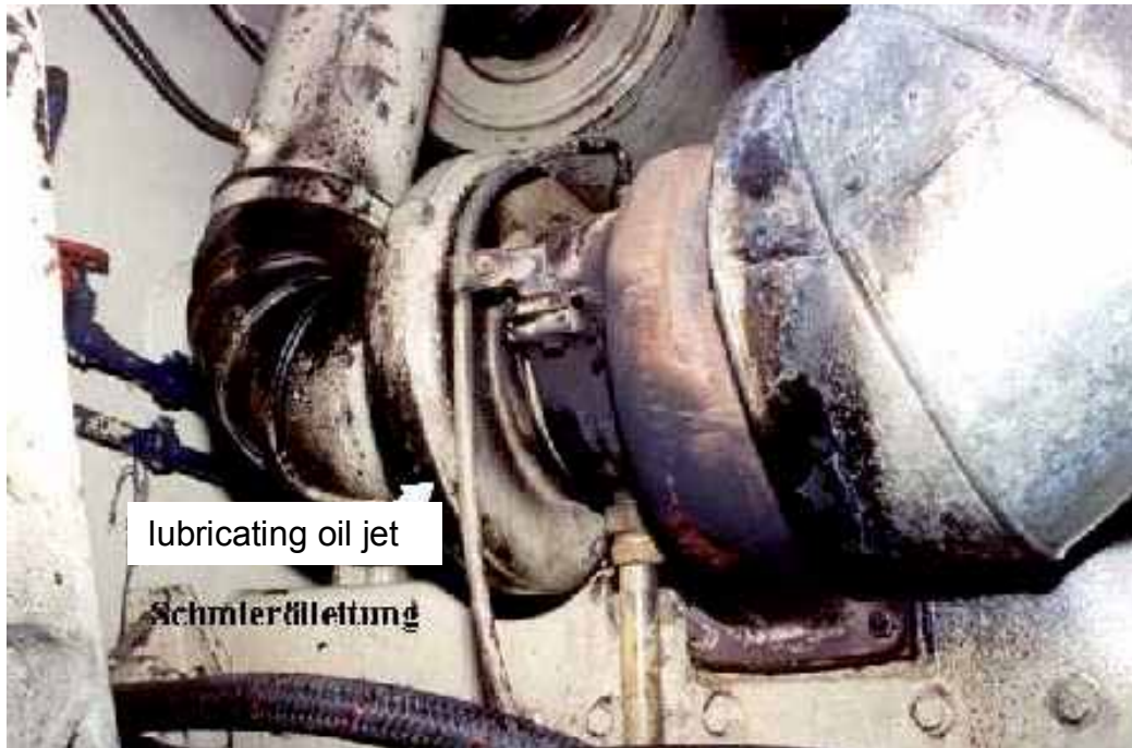
Figure 14: Exhaust gas turbocharger insulation removed
