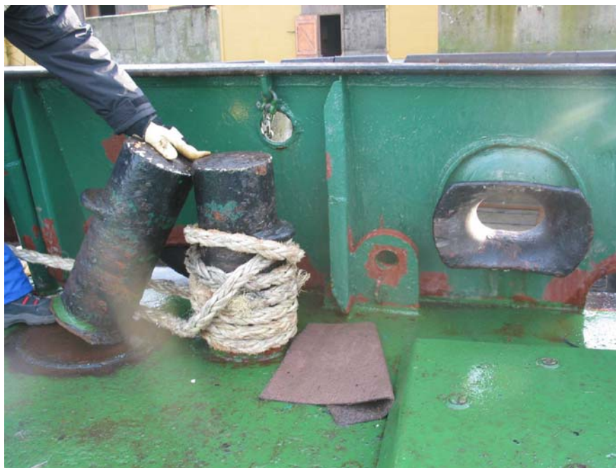
Figure 11: Bollard and hawse
