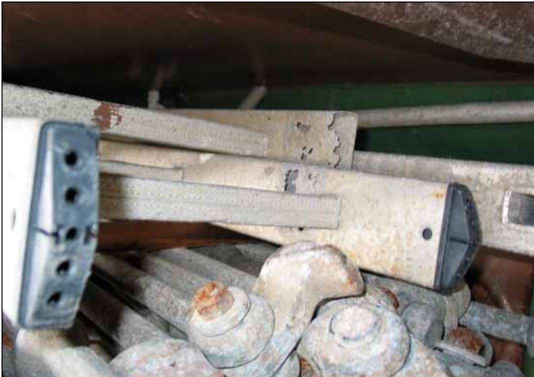
Figure 11: Corroded ladder ends
