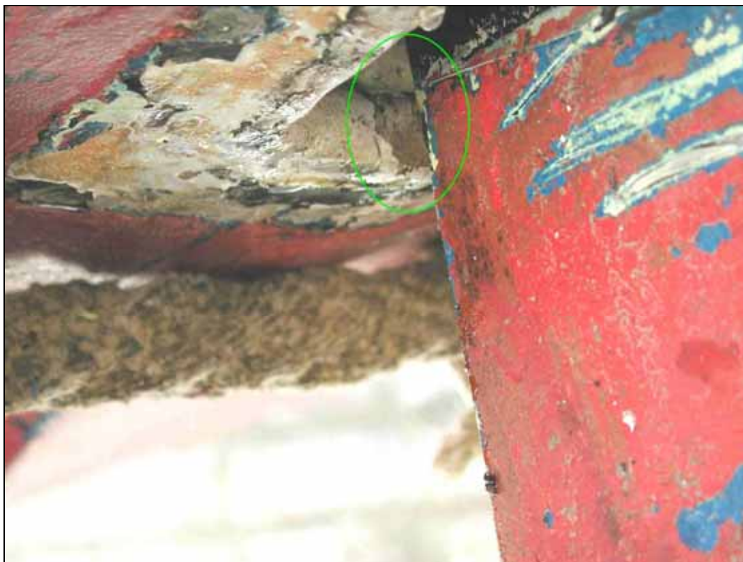
Figure 10: Damage to the trunk of the Saildrive
