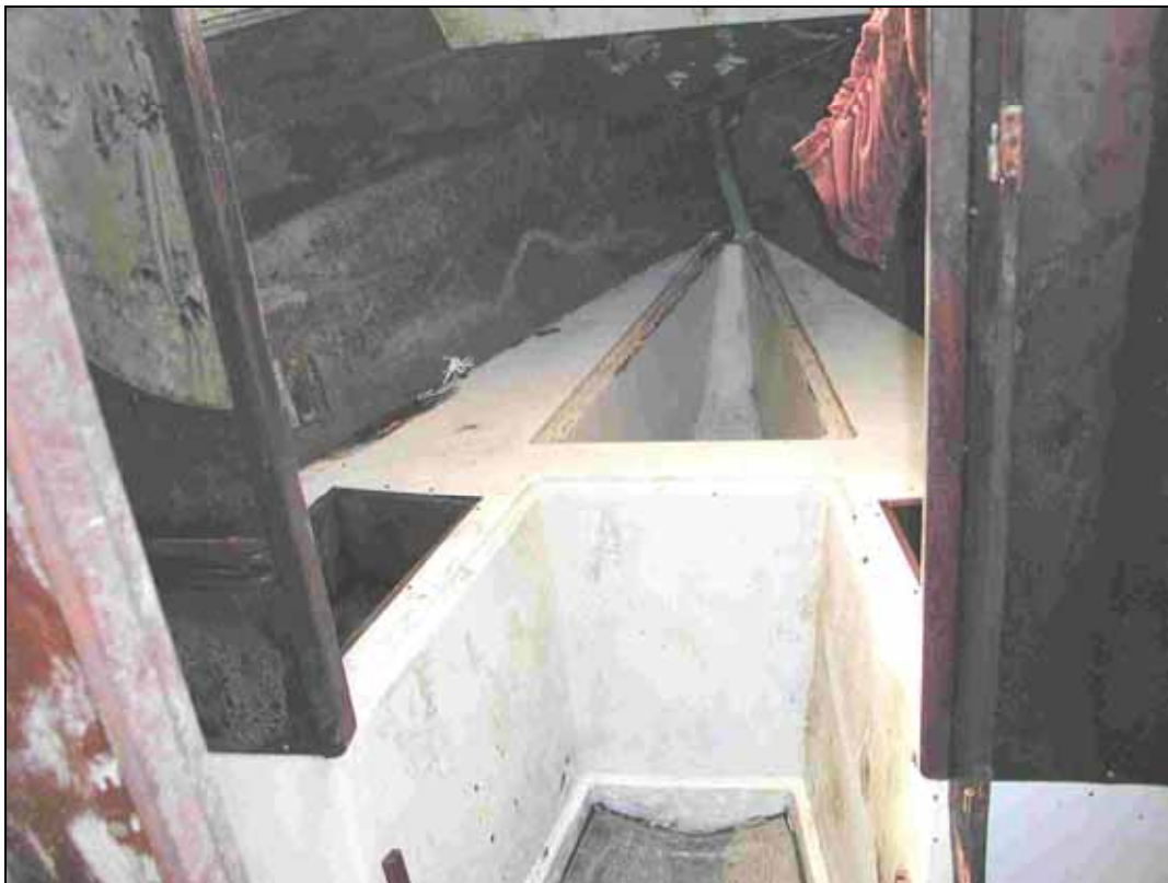
Figure 14: View into the fore ship
