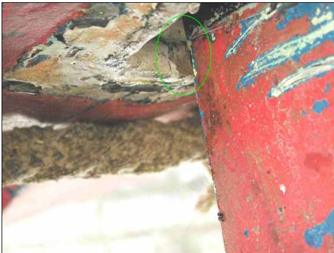
Figure 10: Damage to the trunk of the Saildrive
