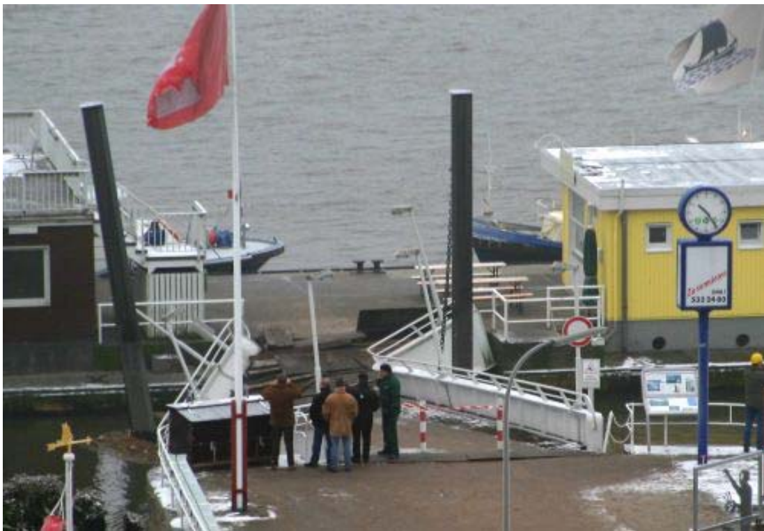
Figure 3: Link span Blankenese
