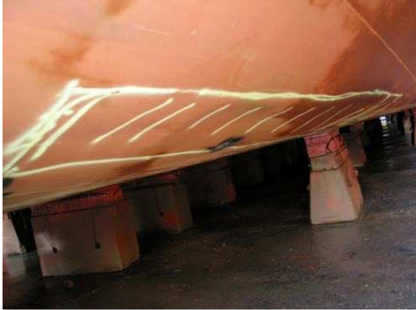
Figure 6: Bottom damage ILKA
