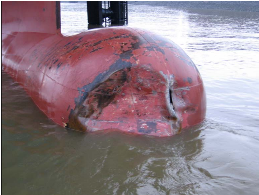
Figure 5: Damaged Bulbous Bow of NYK ESPIRITO
