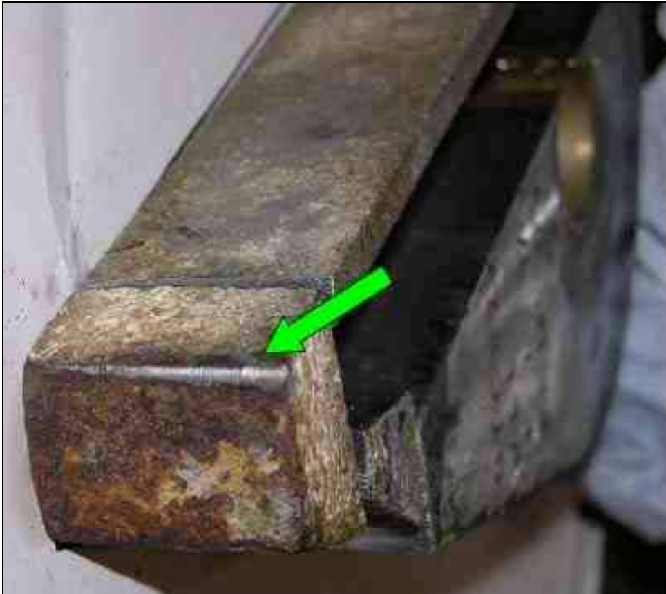
Figure 25: View of the forward hook; asymmetrical rounding, wear edges, strong corrosion
