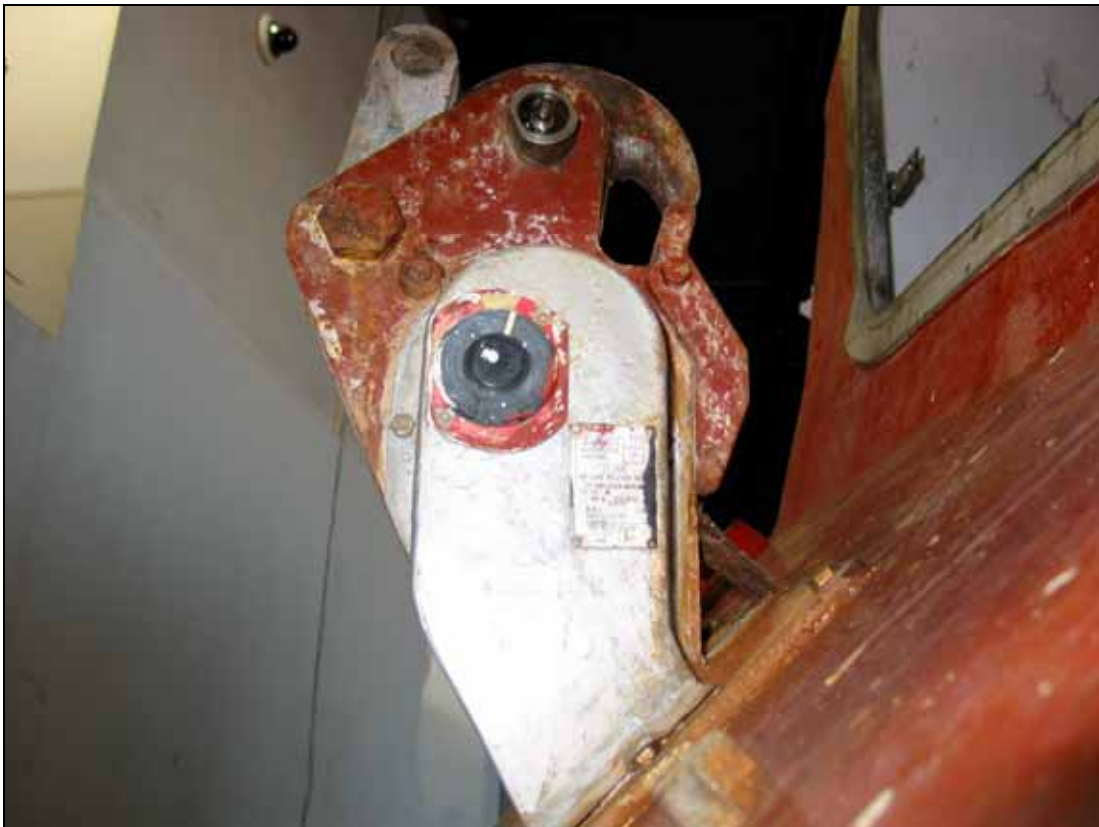
Figure 15: Aft releasing hook, starboard side, with renewed cover
