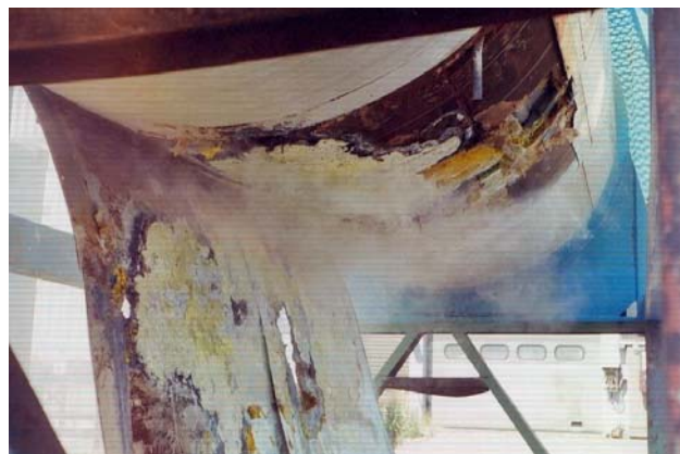
Fig. 5: Removal of the insulation
