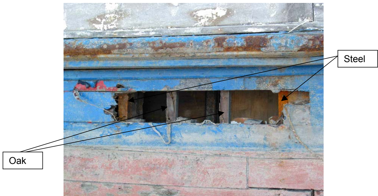
Figure 7: Construction method frames/planks
