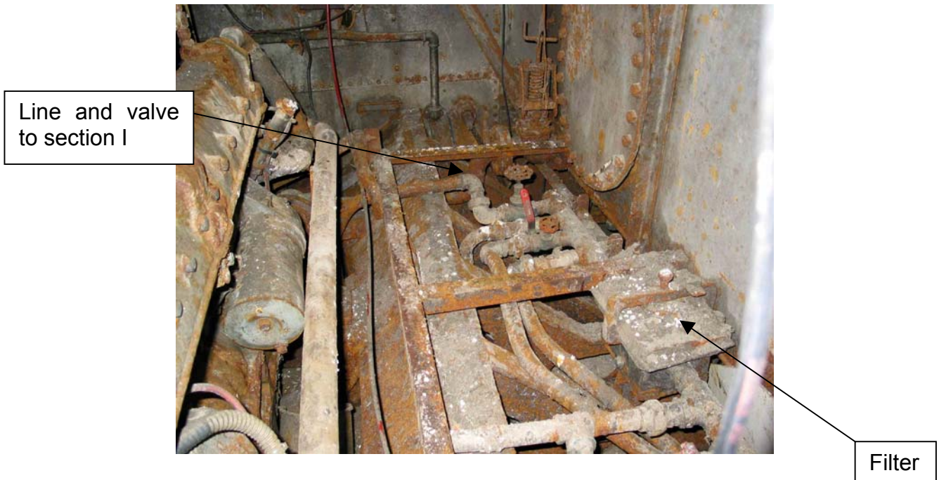
Figure 13: Valve assembly
