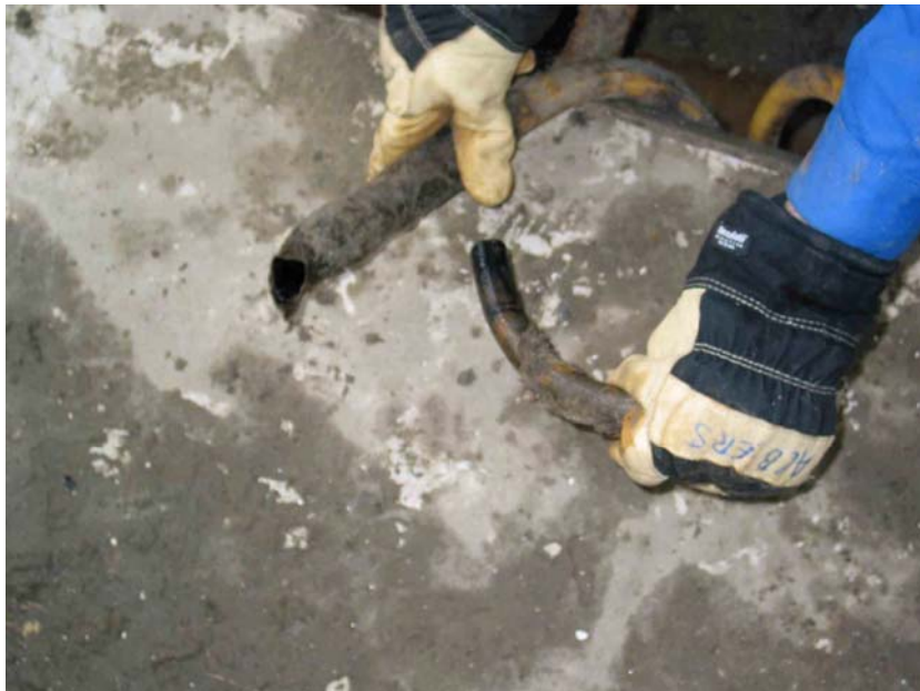
Figure 17: Loose hose connection
