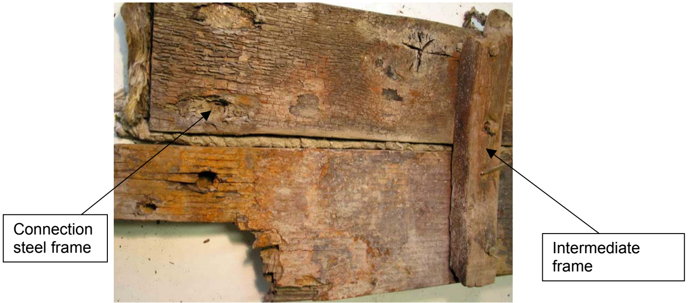
Figure 8: View of planking, interior
