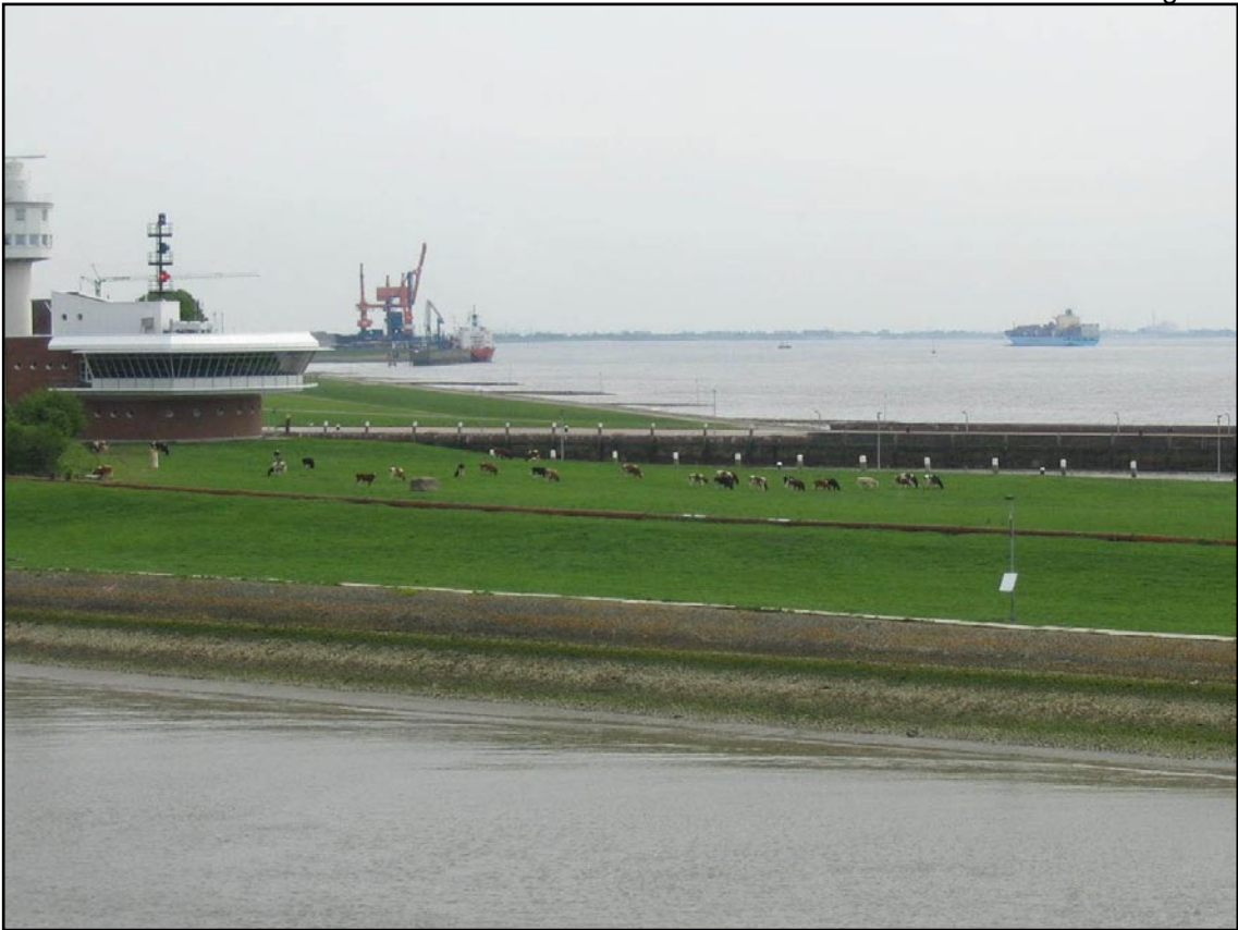
View east by day from bridge of Arctic Ocean in exit basin from Brunsbüttel Lock
