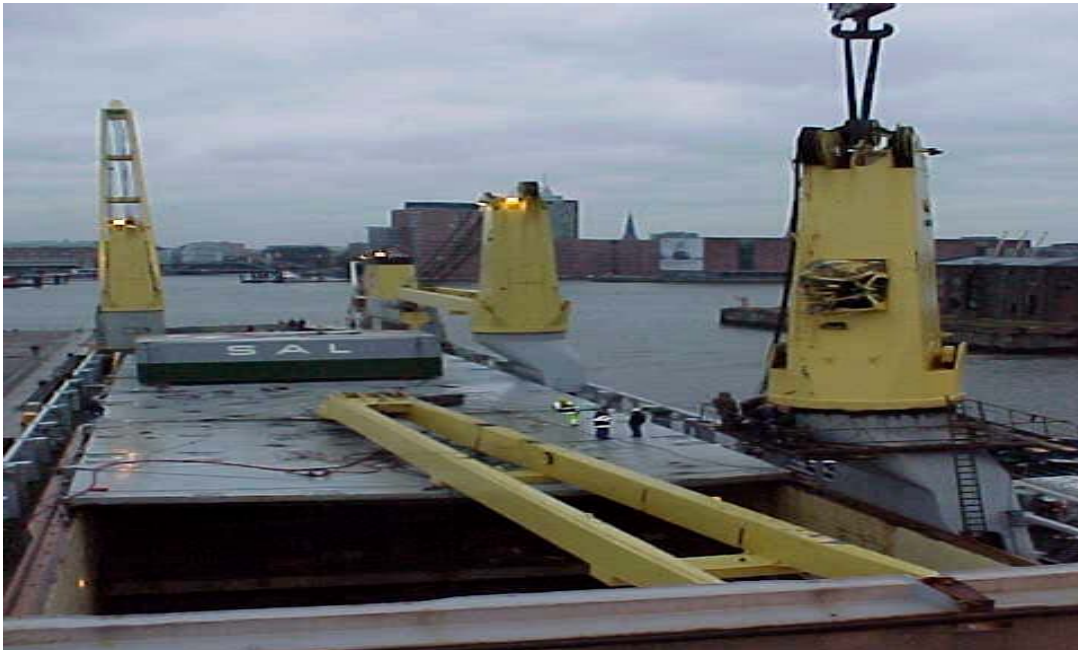
View from the bridge to the aft: the torn off derrick on the hatch cover
