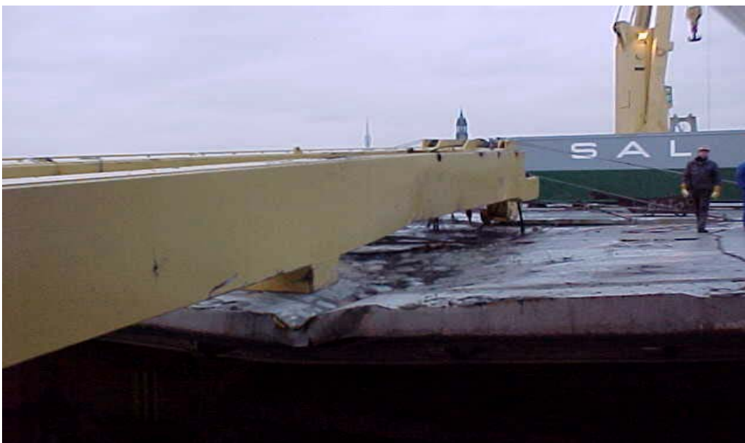
The damage caused to the hatch cover by the fallen crane leg
