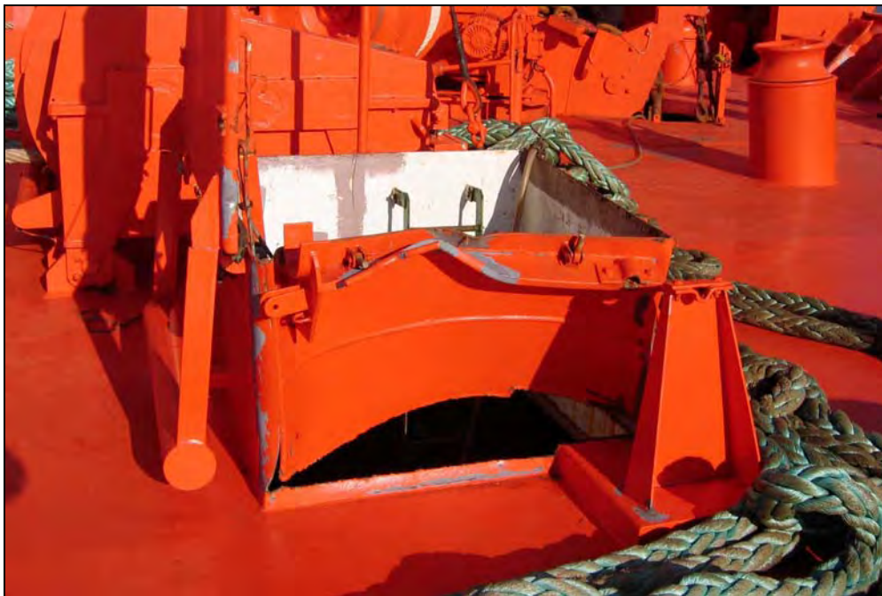
Figure 4: Damaged hatch entry on the forecastle
