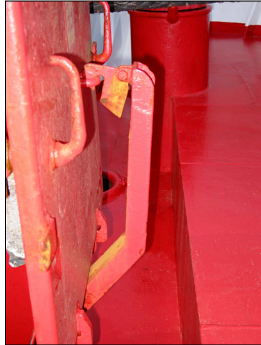
Figure 5: Intact device (No 2)
