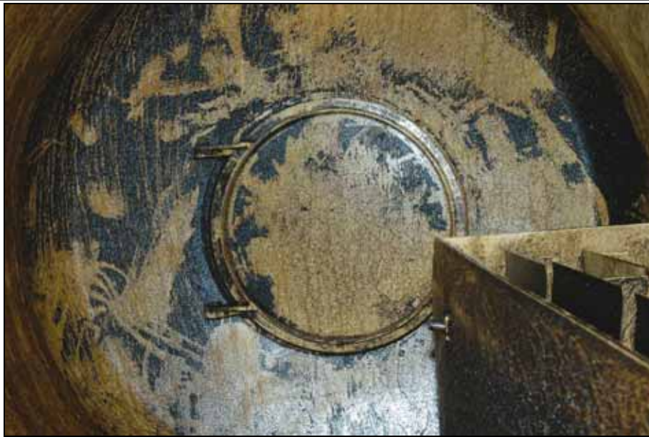
Figure 22: Scavenge air receiver manhole cover – forward end – inside view 29
