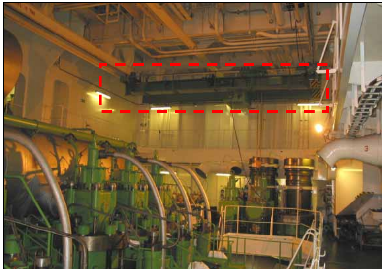
Figure 24: Gantry crane system
