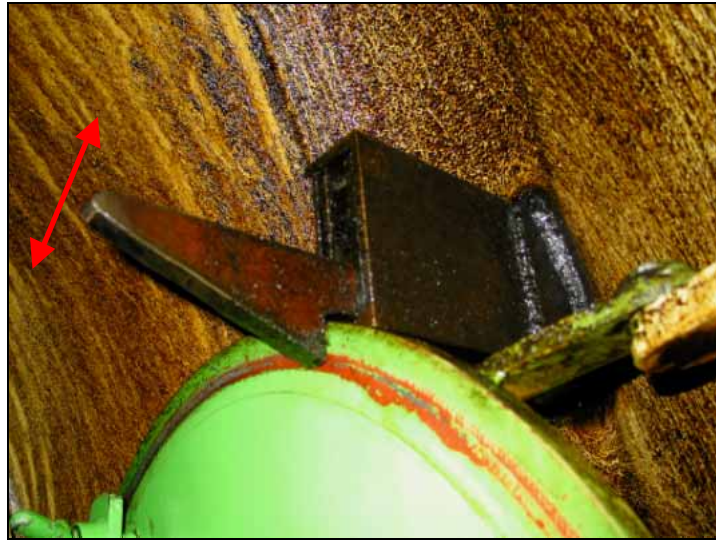
Figure 59: Latching hook fitted and in action
