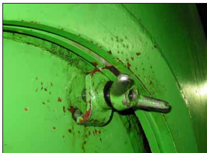
Figure 31: Bolt as a blocking obstacle
