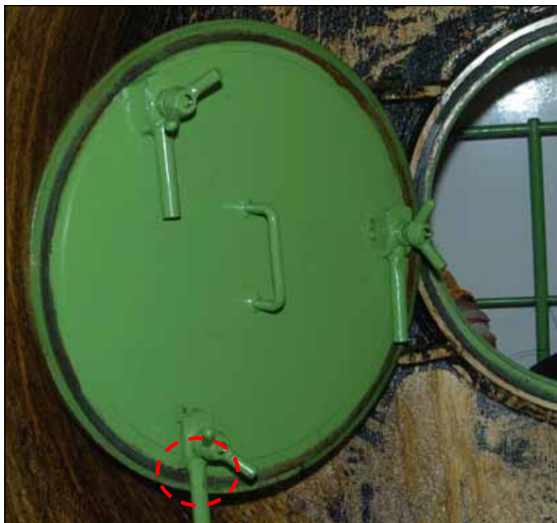
Figure 56: Blocking position of the welded pipe extension
