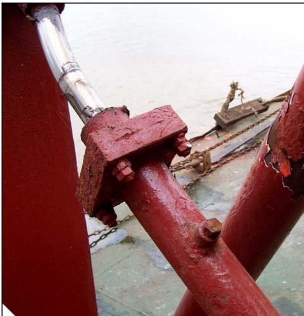
Figure 4: Shock absorber plunger
