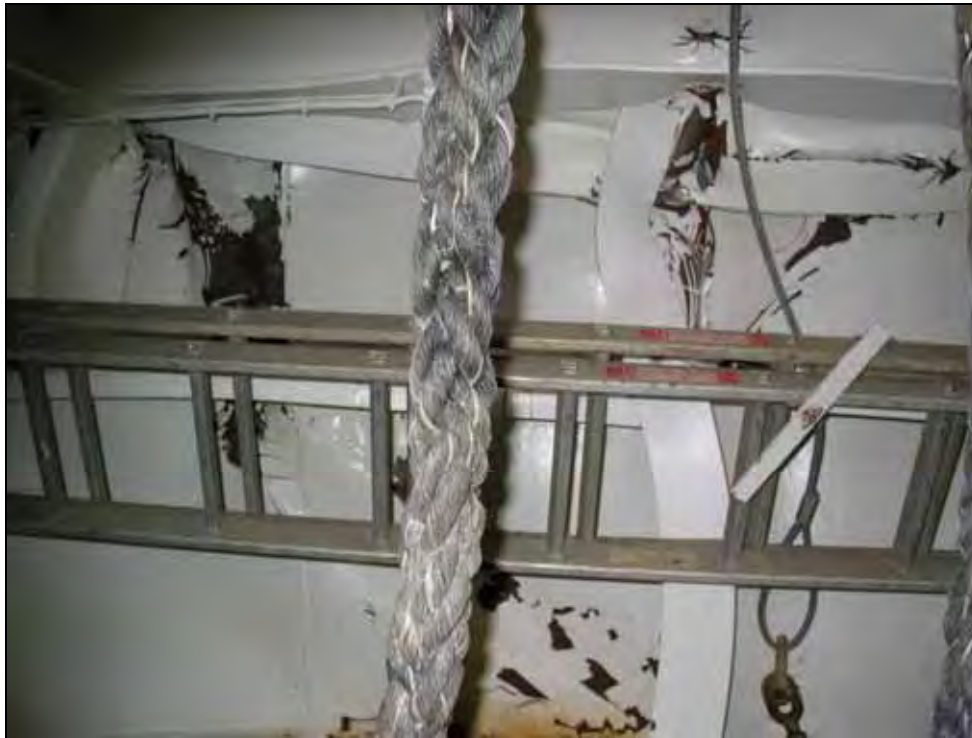
Figure 14: Damage to the interior of the LASS URANUS
