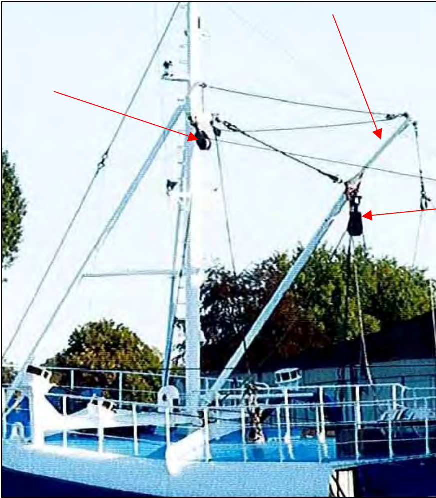
Figure 54: Mast with various pulleys
