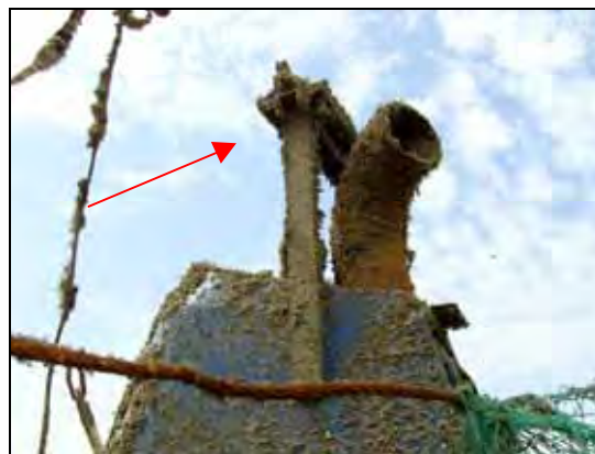
Figure 42: Guiding pulley at the stack
