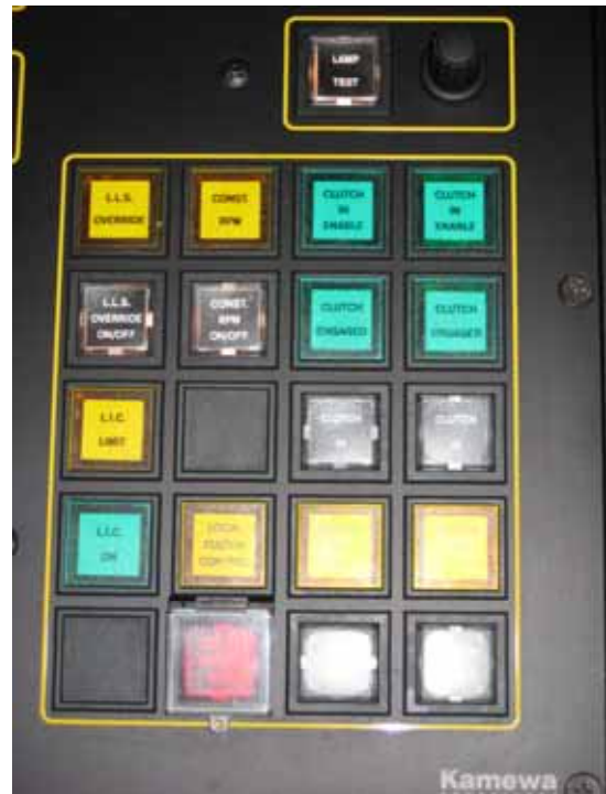
Fig. 6: Bridge wing conning station - load control buttons and indication lamps
