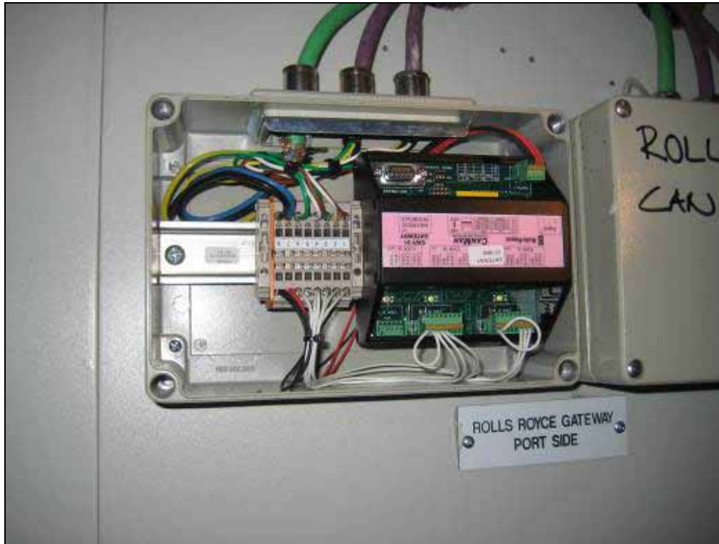
Figure 24: CAN-BUS box on the FINNLADY, open
