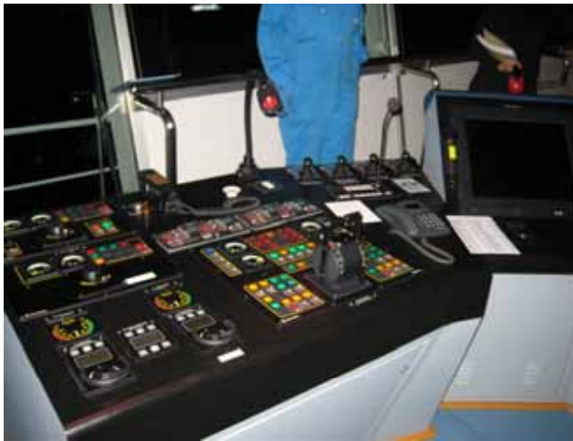
Fig. 1: Bridge wing conning station - overview
