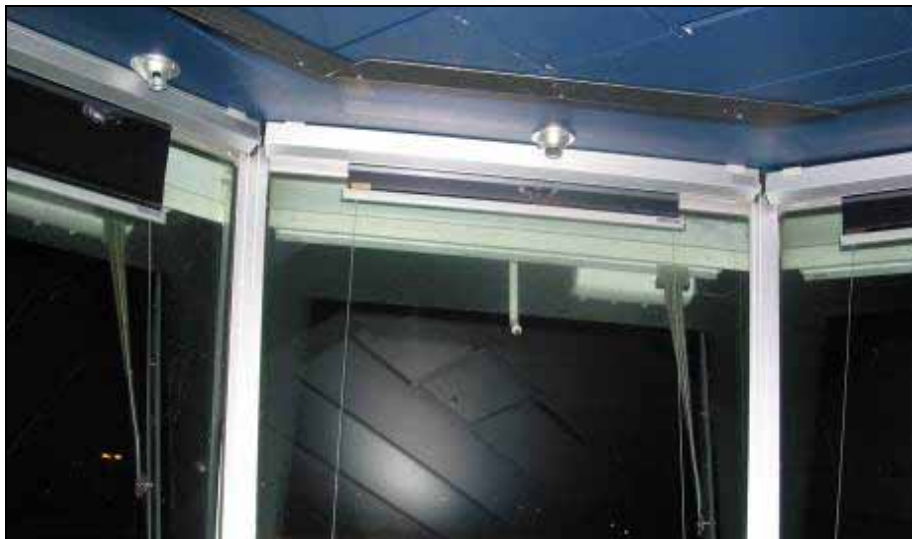
Figure 16: Bridge windows with roller blinds
