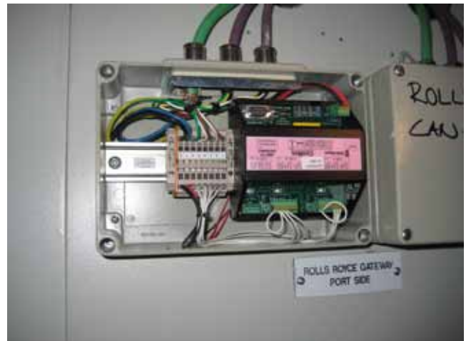
Fig. 16: CAN-BUS housing (opened-up)
