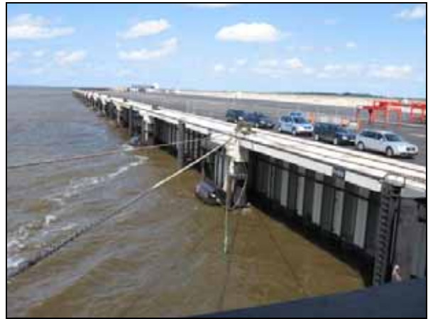
Figure 7: Broken Stern Line
