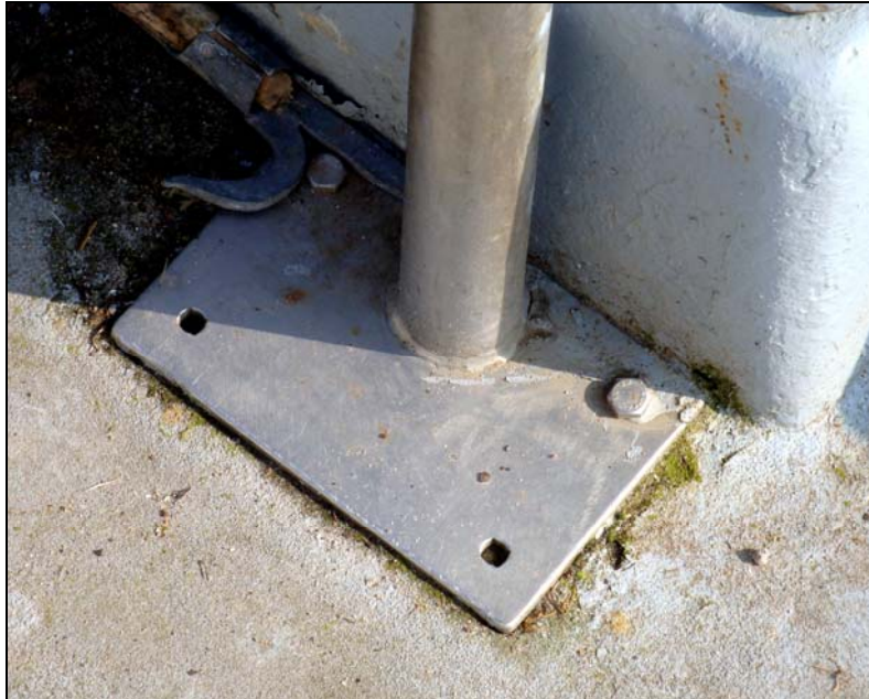
Figure 8: Foundation plate of the starboard mast support
