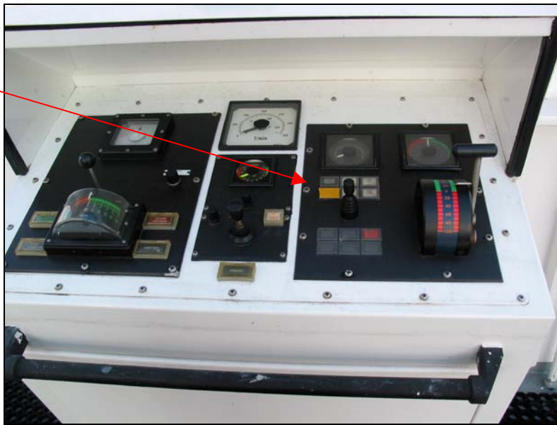
Figure 14: Port bridge wing conning position
