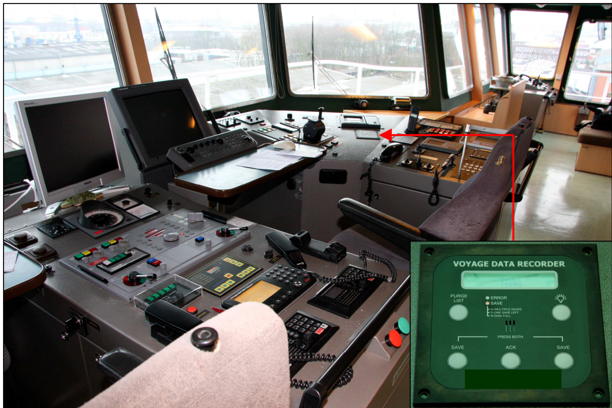
Figure 11: S-VDR control panel in the bridge console
