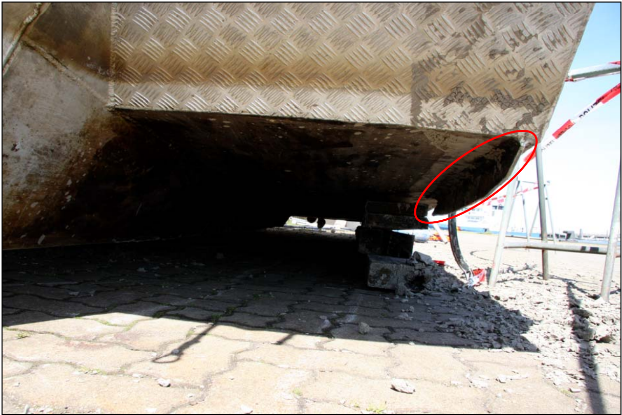
Figure 9: Hull, port side with ballast and forward bilge keel
