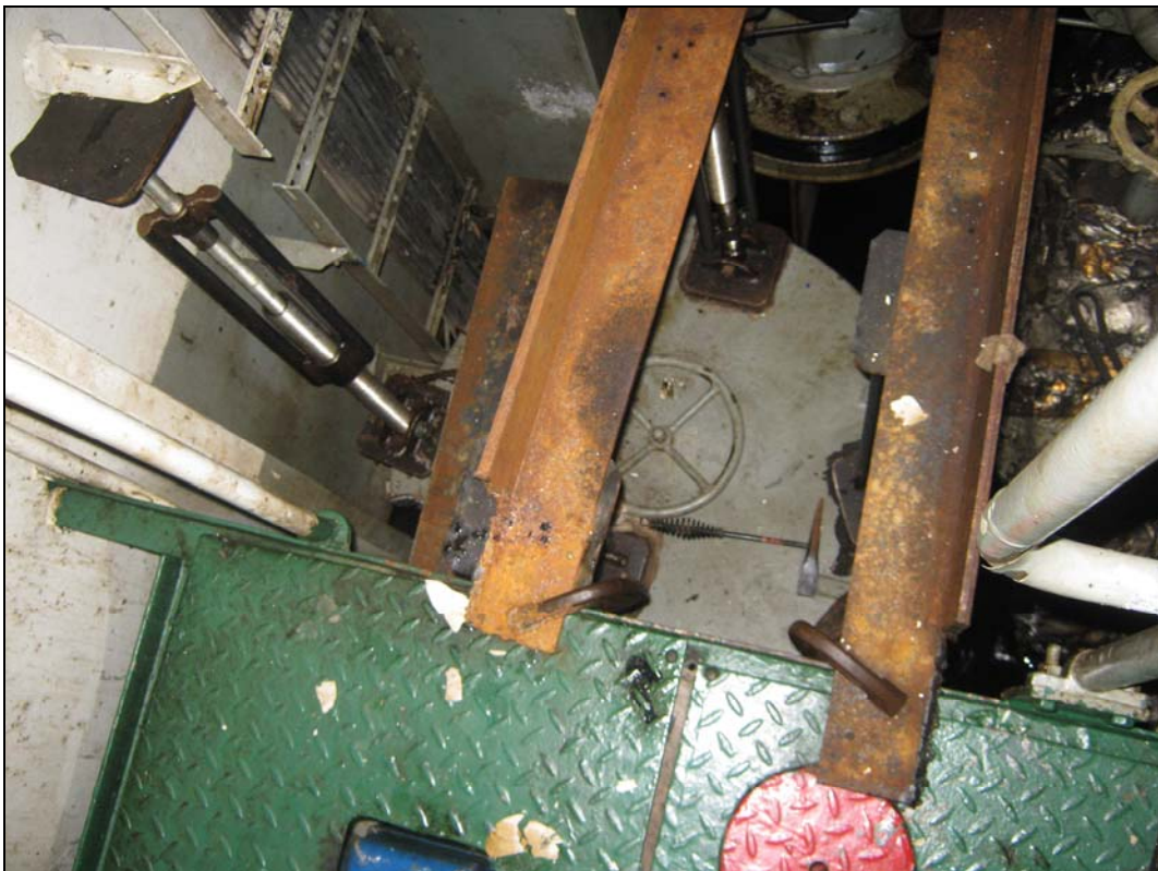
Figure 18: Pipe tunnel cover locked in place
