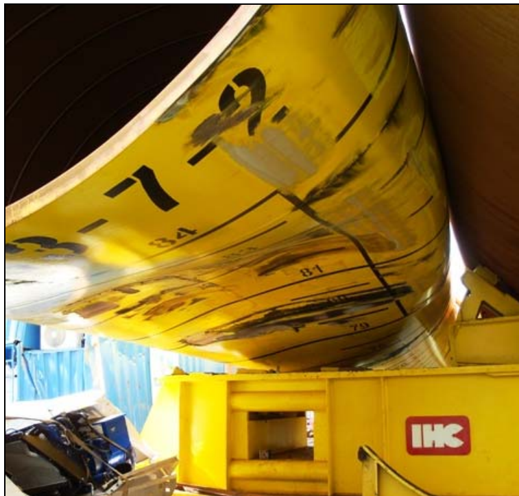
Figure 9: Deformed pile (from below)
