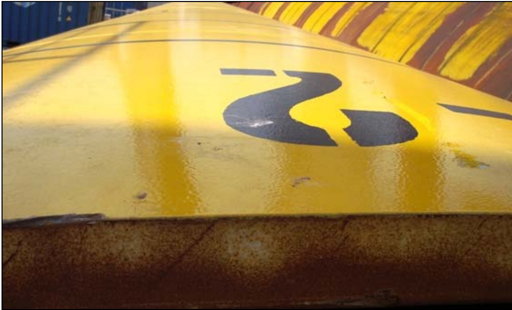
Figure 20: Outer surface of the pile (no pressure marks)
