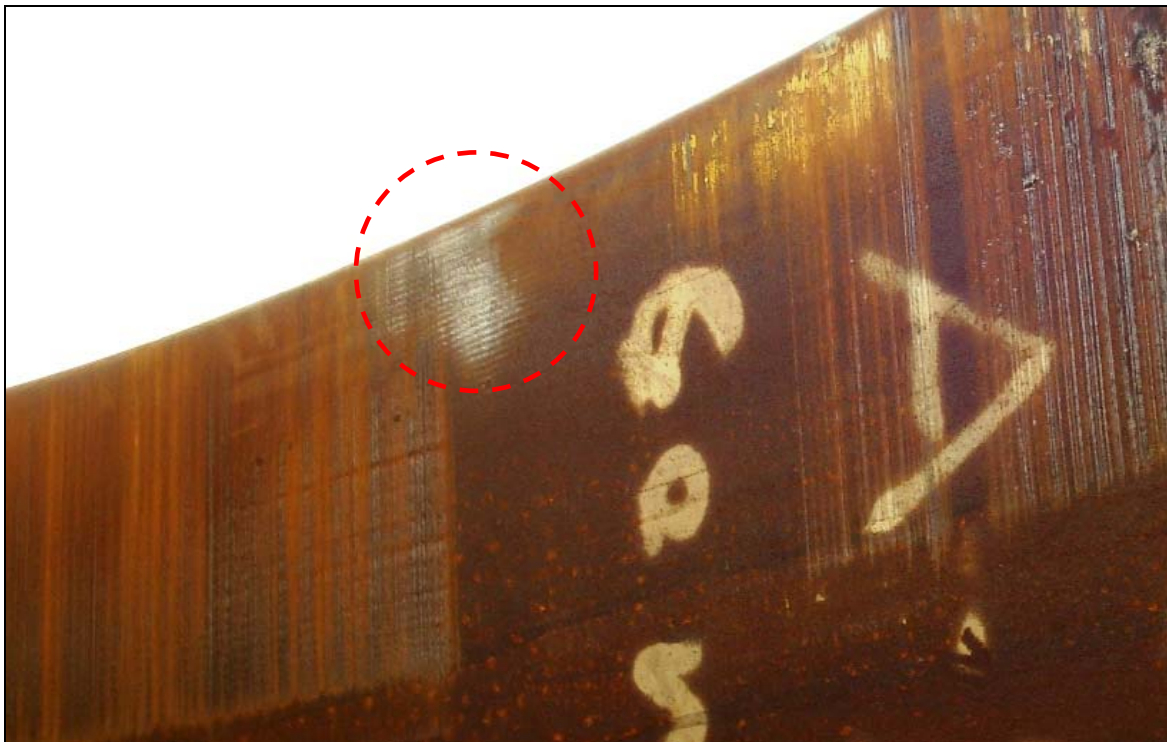
Figure 19: Clamping jaw pressure mark (inner surface of the pile)
