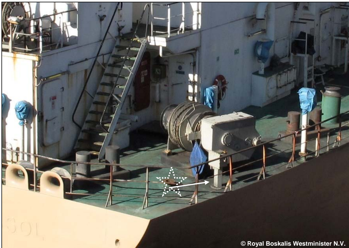
Figure 12: Old and new position of the control unit of the winch 17
