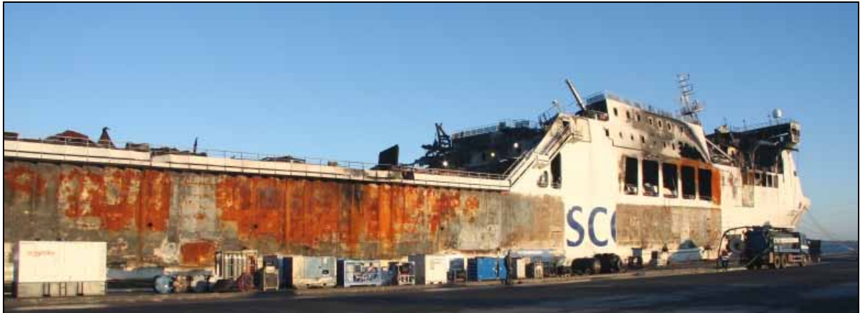
Figure 13: LISCO GLORIA alongside the pier in Munkebo after the fire
