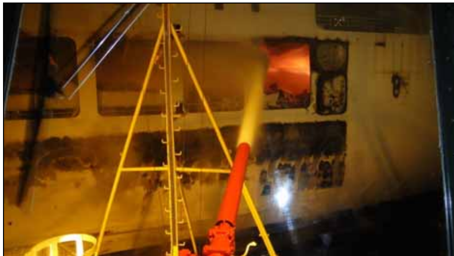
Figure 104: Development of fire damage to the side of the vessel, taken on 9 October 2010 at 0434
