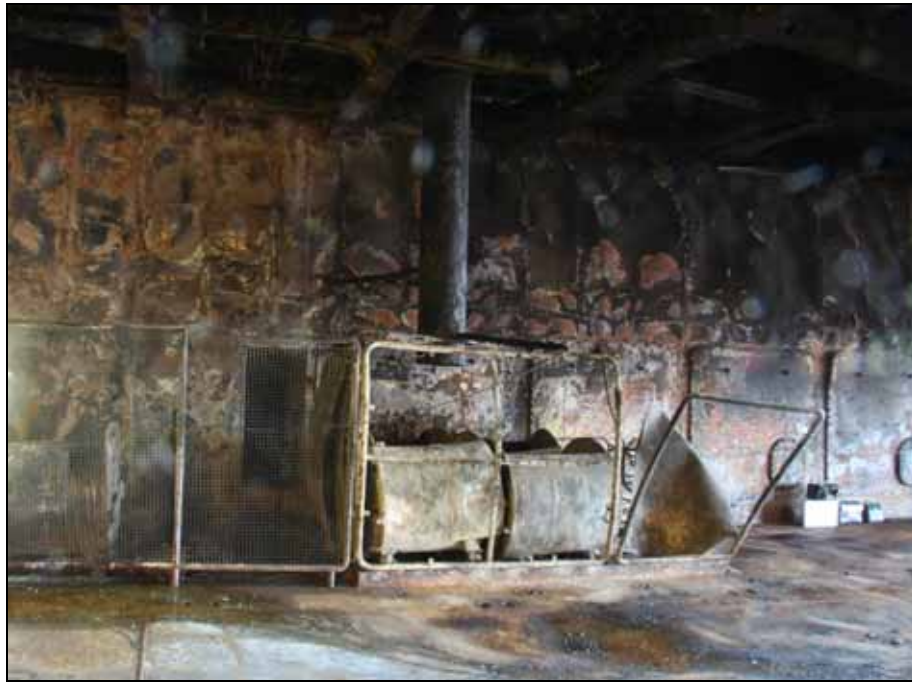
Figure 63: Waste containers and chute on deck 6 after the clearing work
