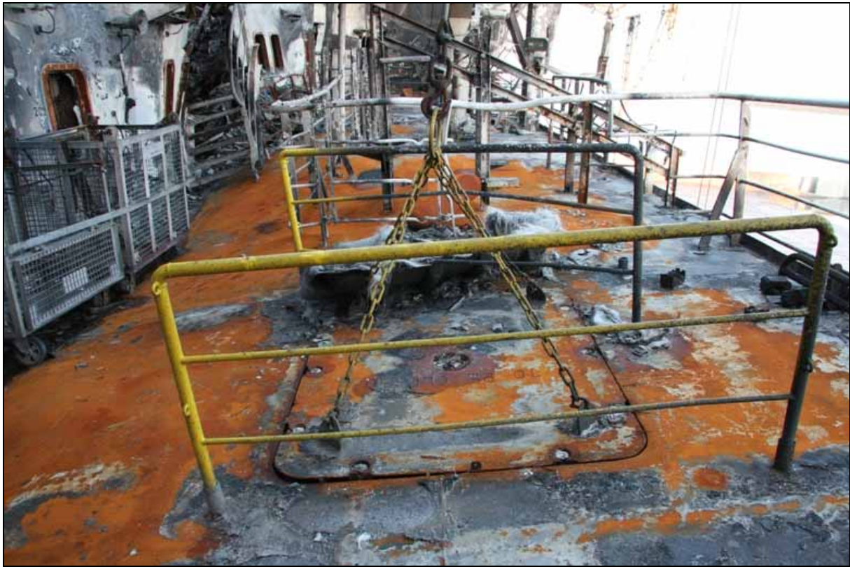
Figure 66: Hatch opening on deck 7 – after the accident
