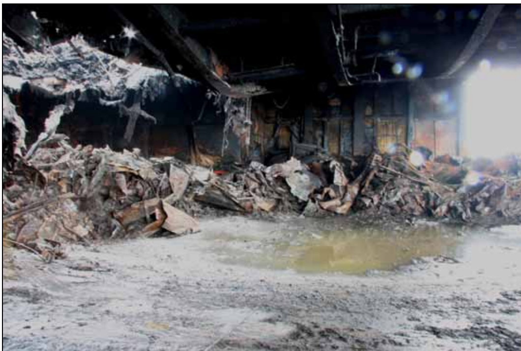
Figure 31: Partly cleared deck 6, view of lanes 5 to 8 in the forward area
