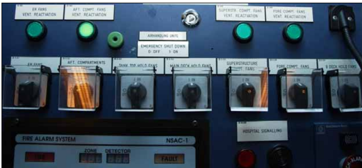
Figure 72: Comparable emergency shut-down for the ventilation system on the DANA SIRENA
