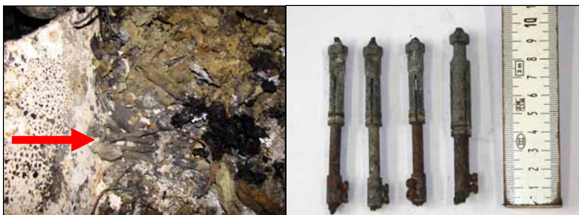
Figure 41: Remains of the male plugs and female contacts from the electrical socket at frame 200 (starboard) 16
