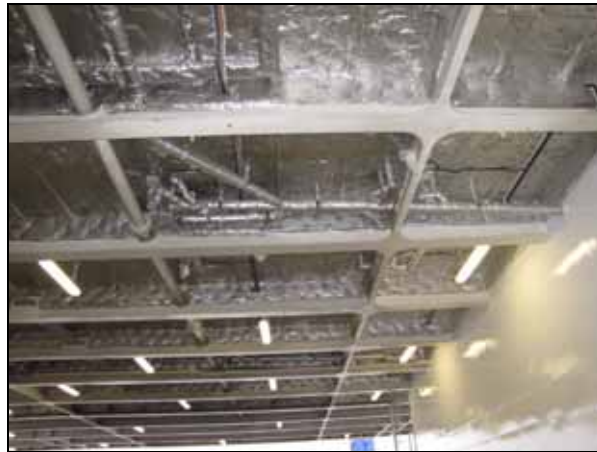
Figure 119: Ceiling covering on the sister vessel, DANA SIRENA
