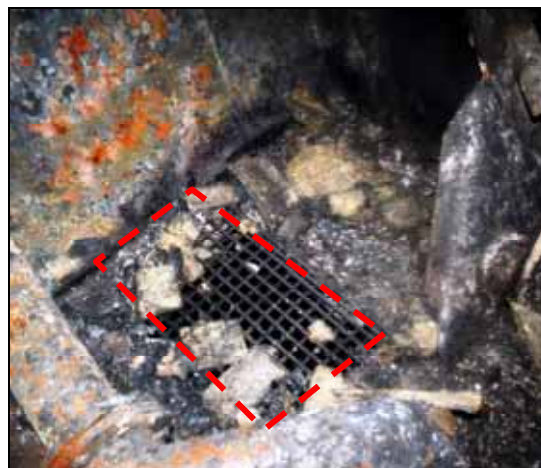
Figure 46: Scupper on deck 4
