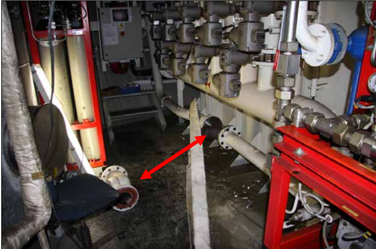
Figure 86: Setup for testing the drencher pump in the sprinkler room
