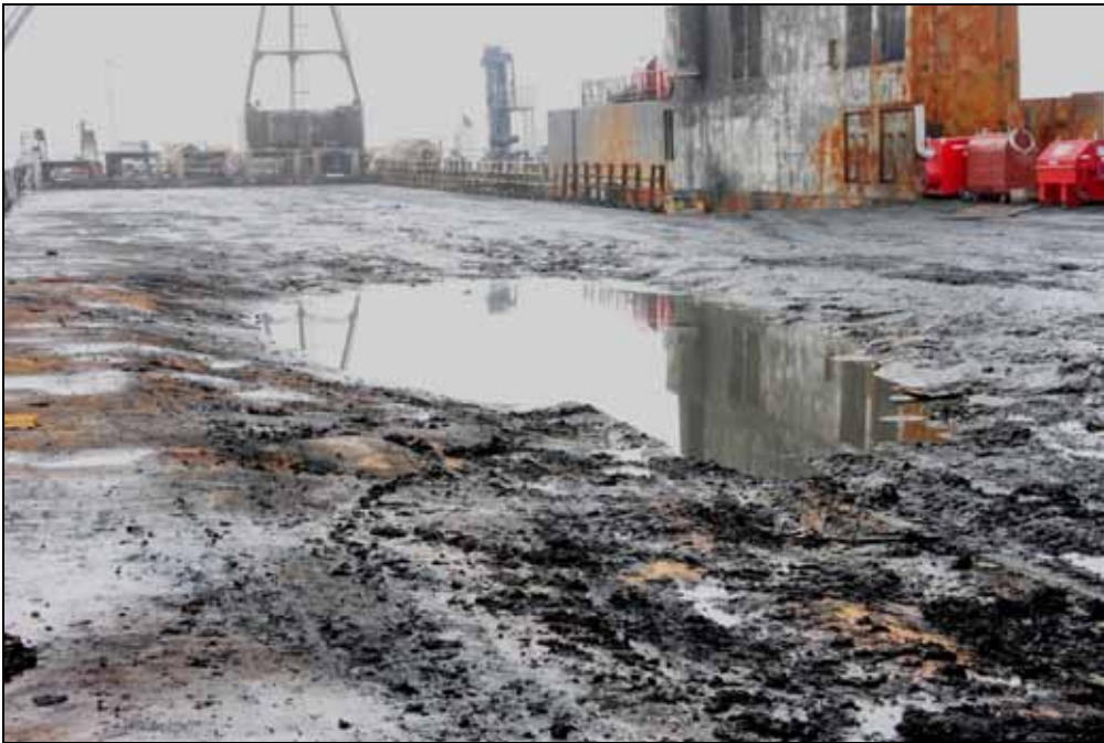
Figure 32: Cleared upper deck (amidships), view to the stern
