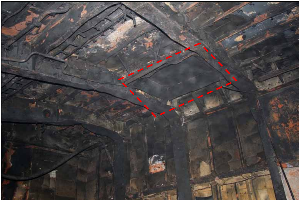
Figure 67: Hatch opening above the first parking position on lane 8 (upper deck)
