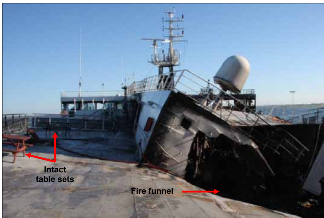
Figure 18: Outside area on deck 9, view to the bow
