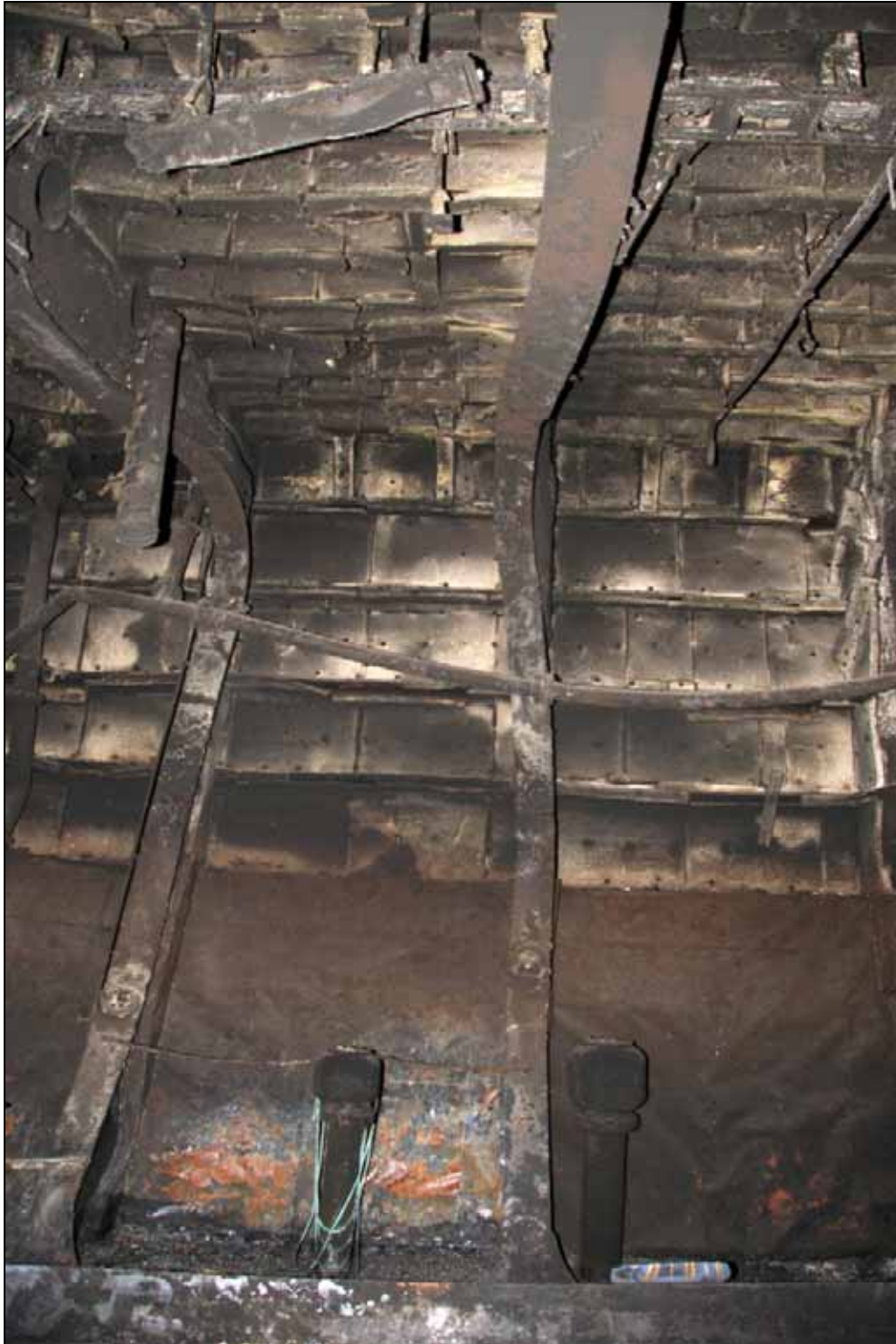
Figure 59: Remains of the A-60 insulation on deck 4
