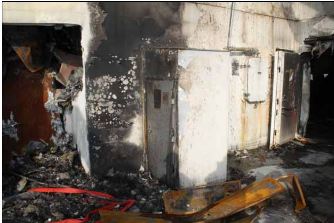
Figure 64: Area outside of the galley, starboard side of deck 7
