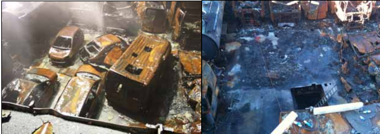
Figure 30: Area on the upper deck cleared for fire-fighting – before and after
