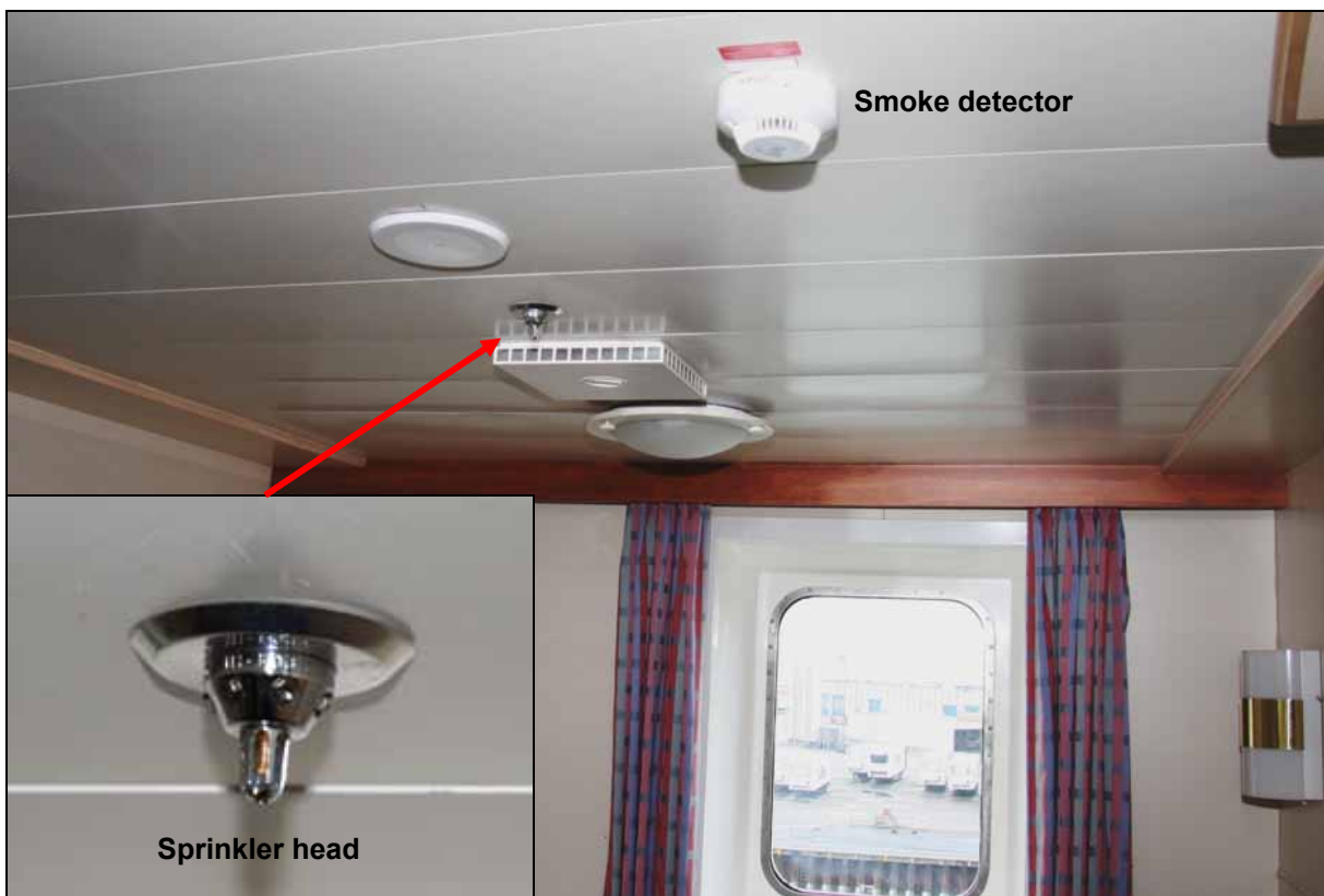
Figure 87: A smoke detector and sprinkler head in a comparable cabin on the DANA SIRENA
