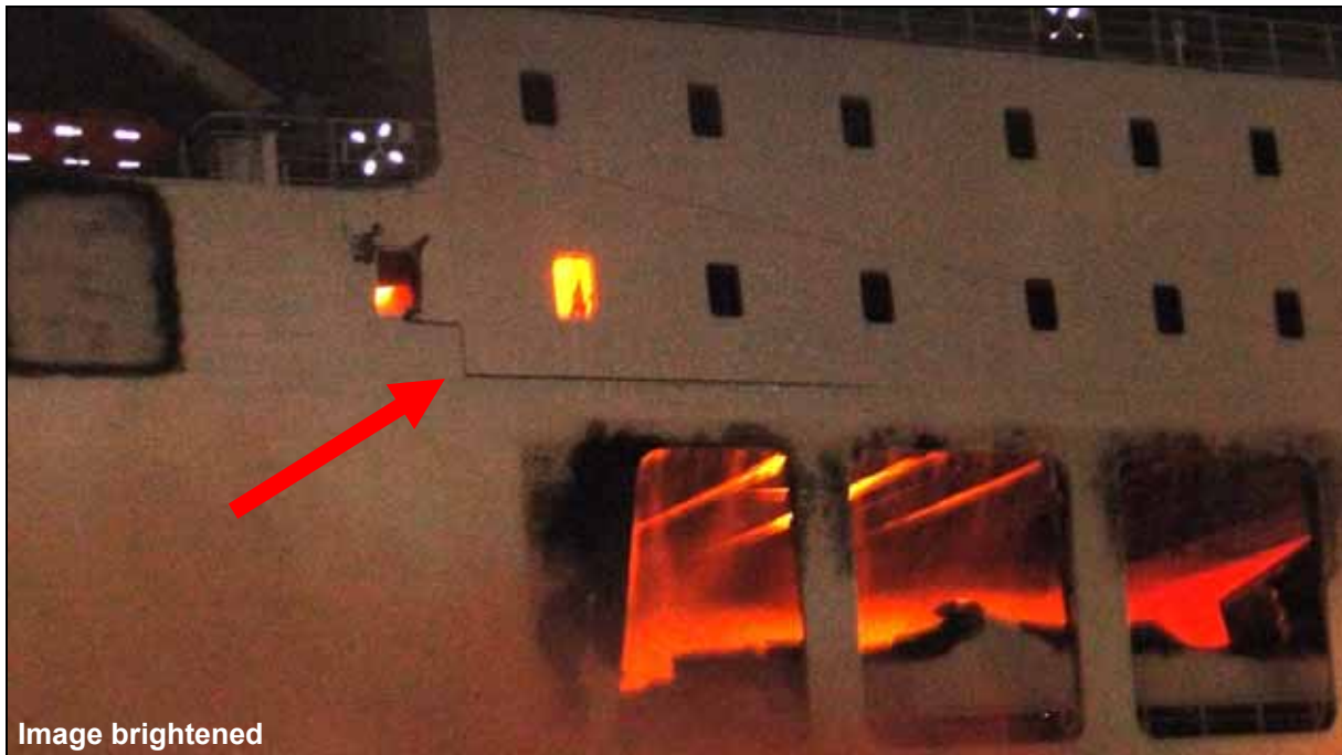
Figure 106: Crack forms between decks 6 and 7, taken on 9 October 2010 at 0629
