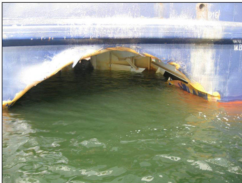
Figure 12: Hole level with the waterline in the shell plate of the URD
