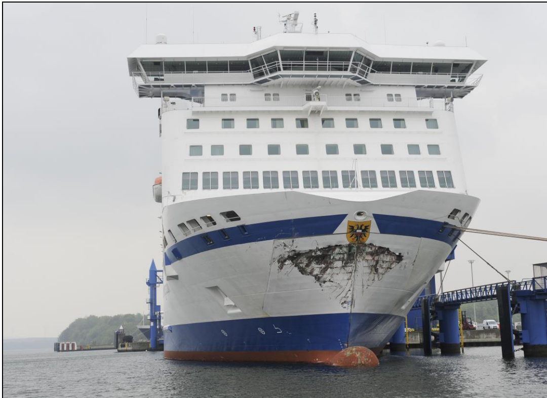
Figure 9: Damage to the bow visor of the NILS HOLGERSSON
