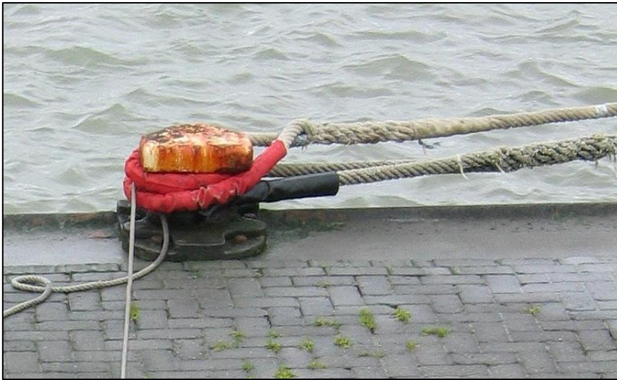
Figure 7: Bollard with two lines placed over it
