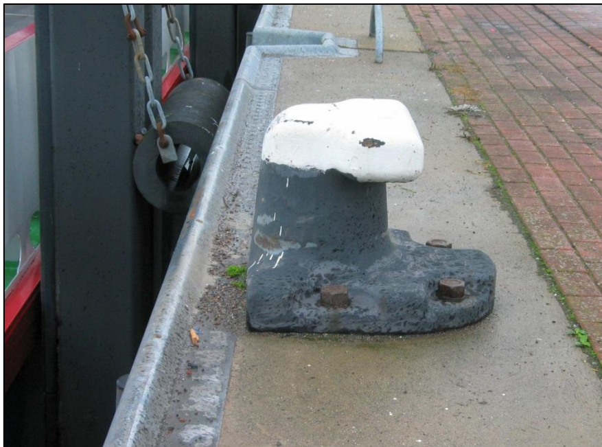
Figure 9: Edge of the quay with bollard, dolphin, and fender
