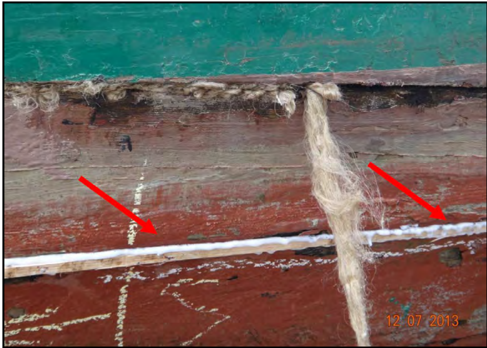
Figure 9: Bonded wood strips in longitudinal joints
