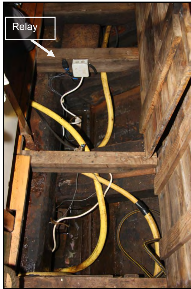
Figure 14: 12-volt pumps, hoses, and electric cables
