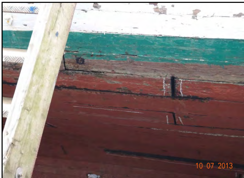
Figure 8: Plank joints
