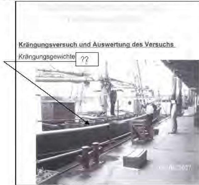
Figure 3: Performance of an inclining test
