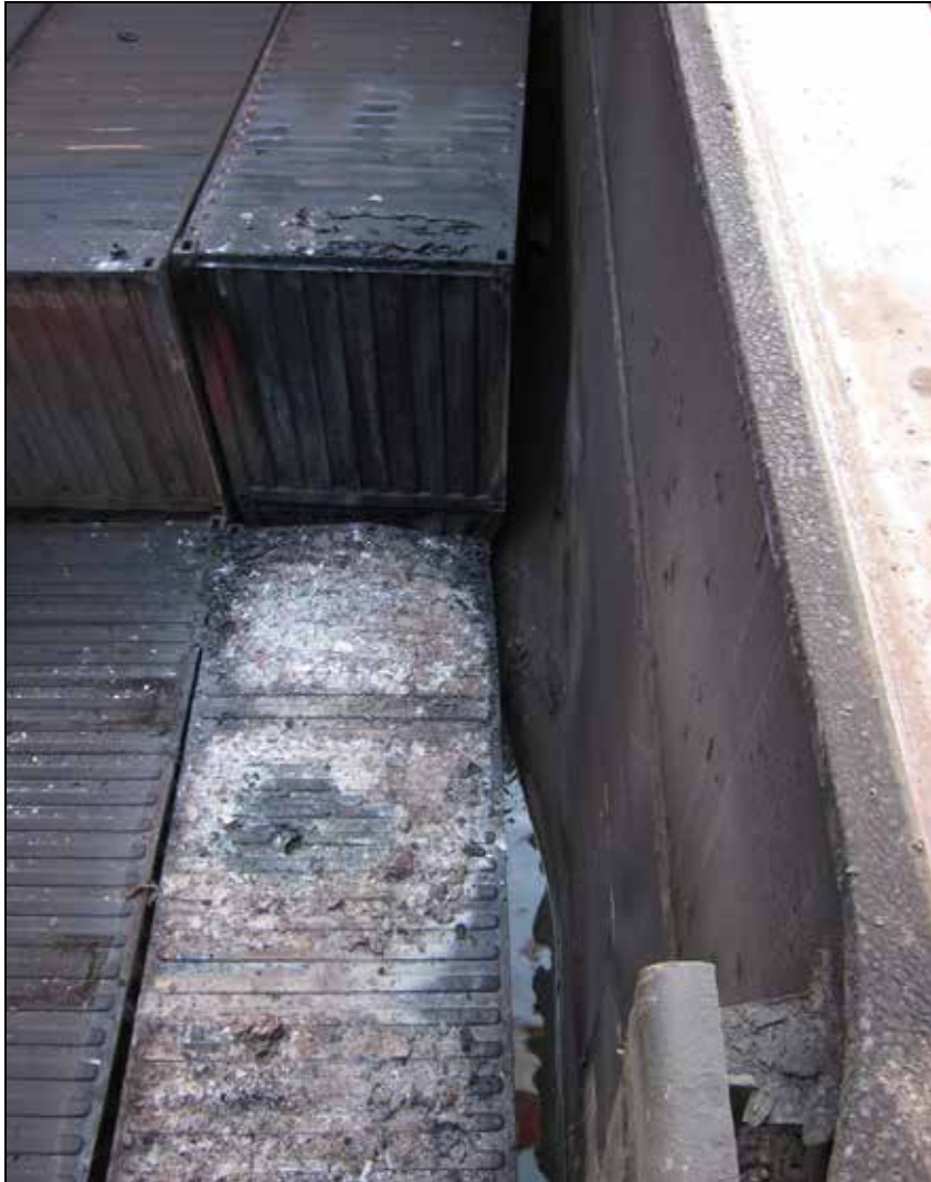
Figure 16: Water ingress and evidence of heat development in cargo hold 5
